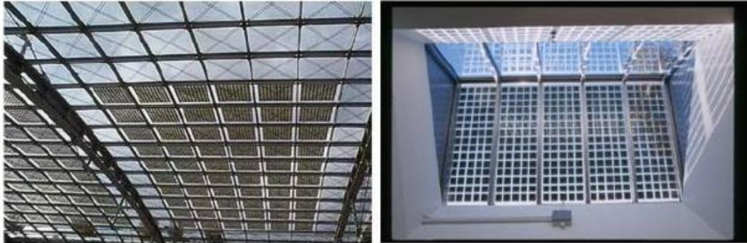
Figure 4.3: Images of integrated PV modules
