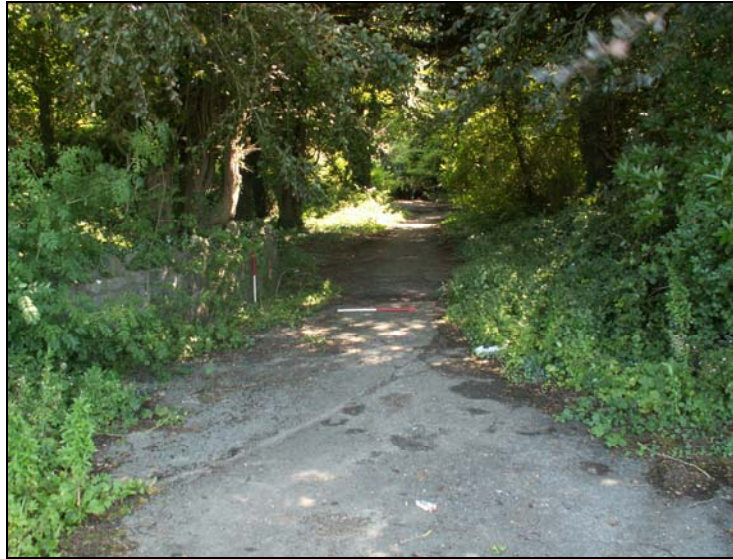
Plate 7: Tarmac driveway leading to Crossways (ID IF09). View to the east.
