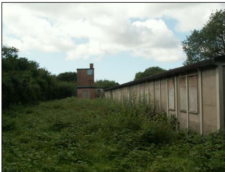
Plate 4: Central boiler room and water tank, Hunt 9 (ID 02215m/31803/LB11362). View to the northeast.
